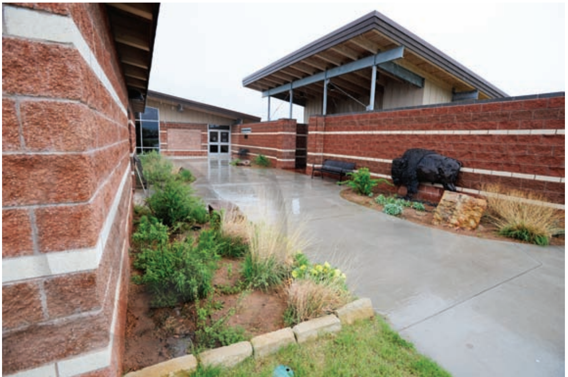
The new park headquarters and interpretive center at Caprock Canyons State Park was built in October, 2007. It is located just three miles north of Quitaque in Briscoe County.
