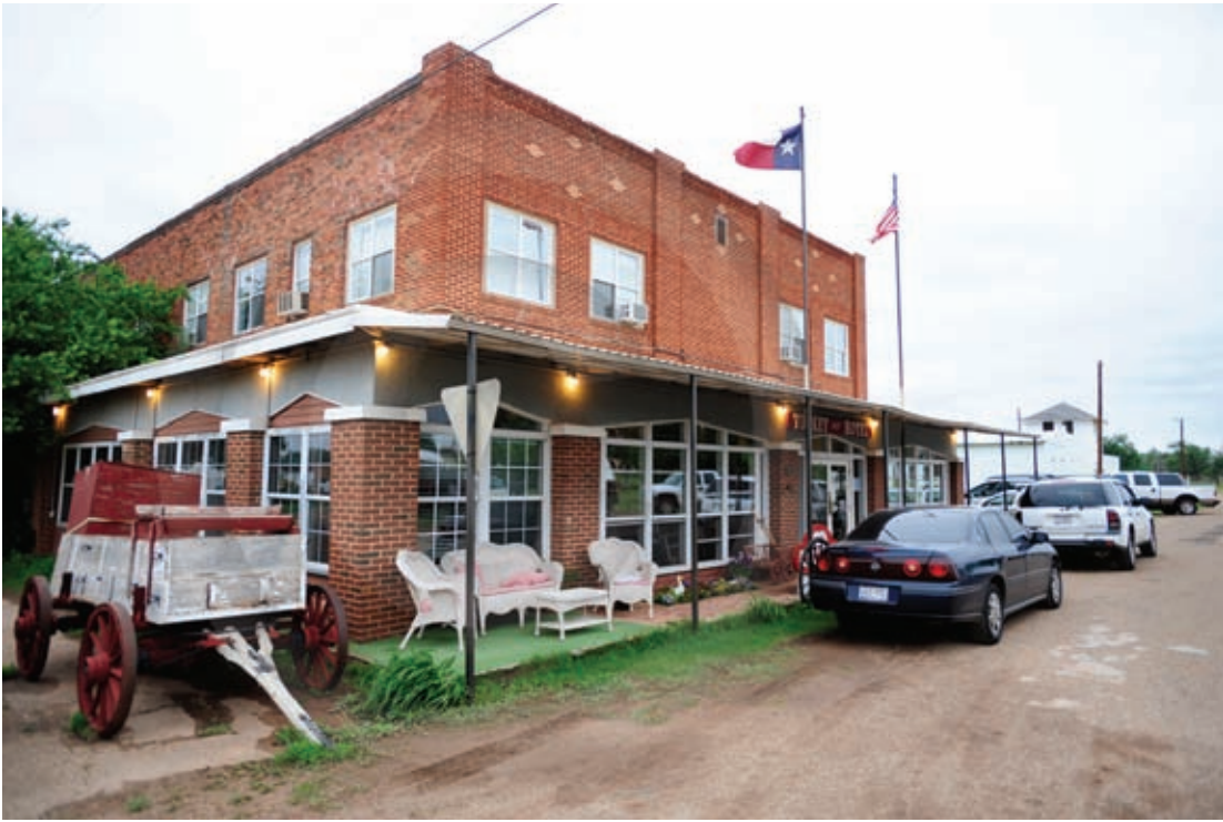
THE OLD HOTEL TURKEY, located just north of downtown in the Hall County town of Turkey, is the hometown of famed fiddle player and band leader, Bob Wills. Few changes have been made in the hotel, which still hosts guests year-round. It is a favorite haunt of those wanting to tour Caprock Canyons State Park.
